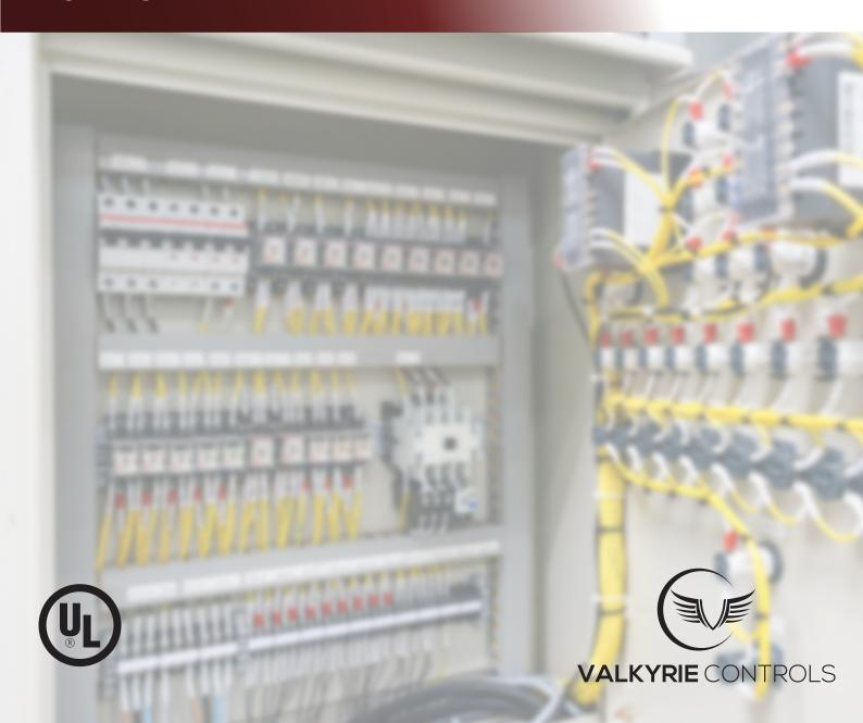
The Halen System is a general-purpose Allen-Bradley based measurement & control panel with 136 channels and equiped with a 17- slot Allen-Bradley ControlLogix PLC.
